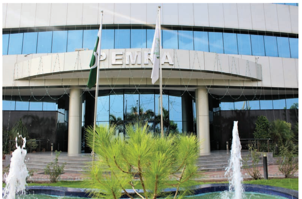
► Illumination of PEMRA Head Office Building on the eve of Independence Day.
